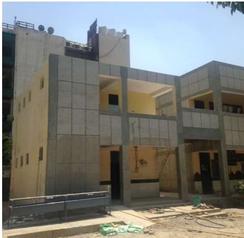
After the upgrade
